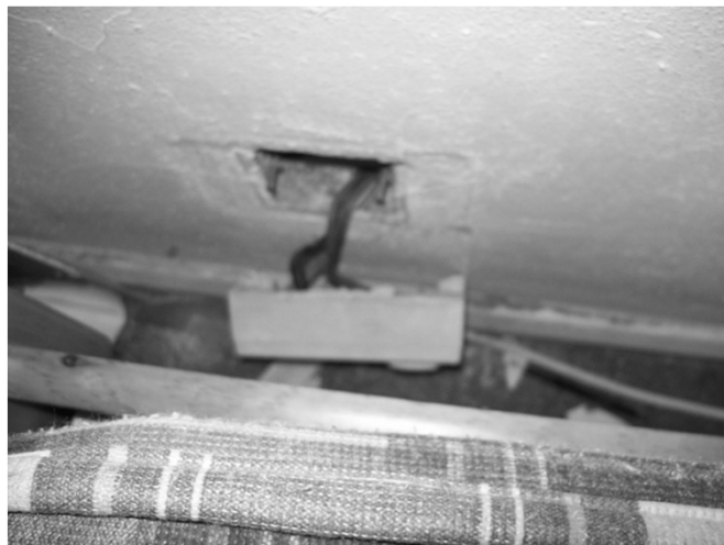
Plug socket behind the same bed with an extension lead on an extension lead
